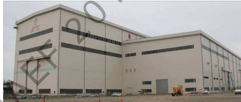
For Reactor vessel / Reactor internal (Futami) under construction
