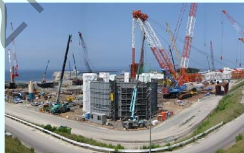
Electric Power Development CO. Ohma-1 (Under construction) (NSSS (Full MOX ABWR))
