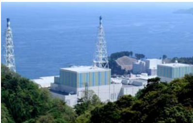
●Chugoku Electric Power CO. Shimane NPS
