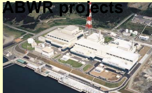
Tokyo Electric Power CO. Kashiwazaki-Kariwa-6/7 (1996/1997) (H/G/T Joint Venture)
