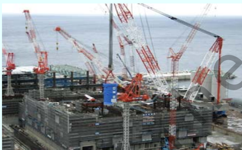
Chugoku Electric Power CO. Shimane-3 (Under construction) (NSSS and BOP)
