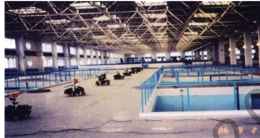
WWTP in China (260,000 m 3 /d)
