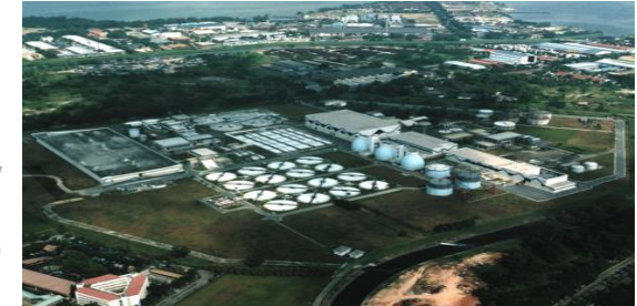
WWTP in Singapore (75,000 m 3 /d)
