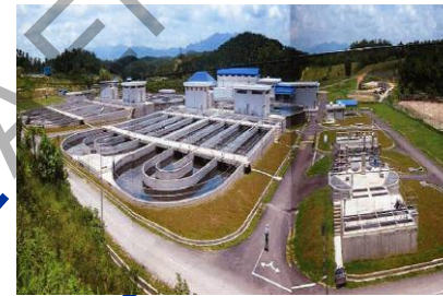
WWTP in Malaysia (59,000 m 3 /d)
